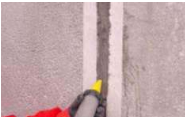
Application of MAXJOINT ELASTIC
