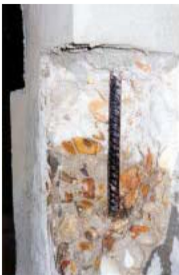
Damp the surface
